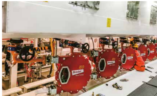
▲ Breidel pumps used for pumping grout between concrete rings and soil
