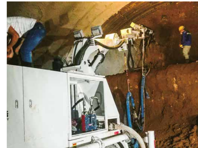
▲ APEX pump delivers accelerator in tough high humidity conditions
