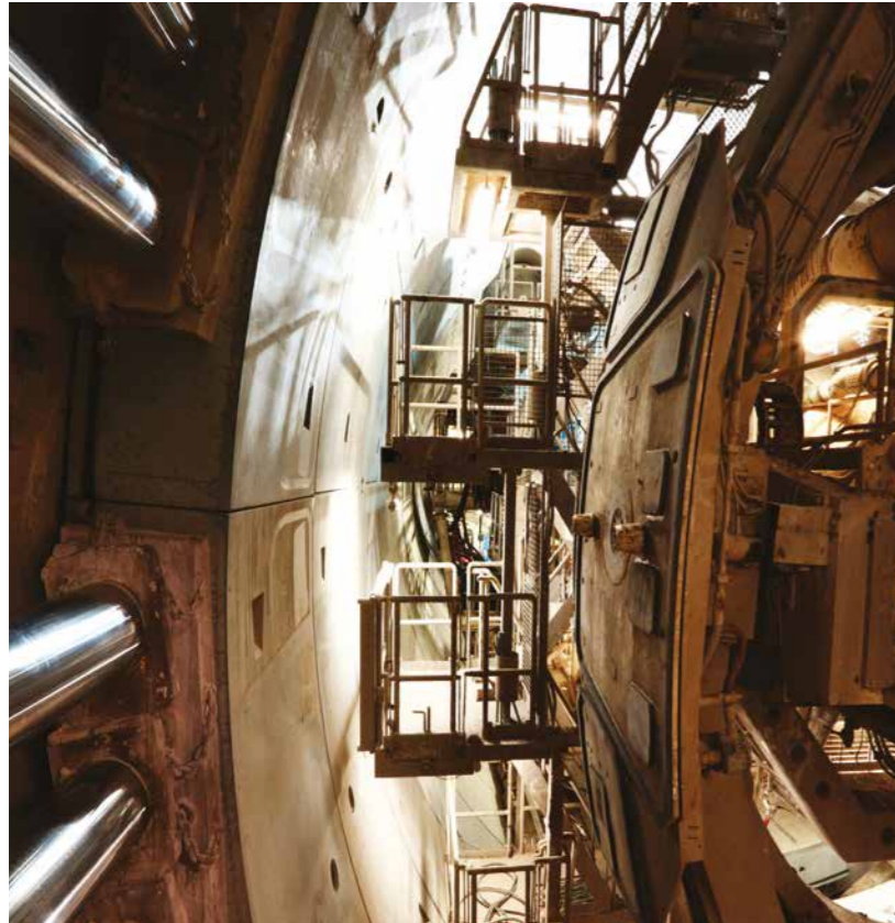
▲ Concrete segments installed to form the tunnel wall
